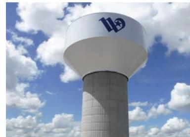
The new, 2 million-gallon Owen Ln. Tower is now complete. The new composite tank replaced the 60-year-old steel tank, improving system redundancy and increasing storage capacity for west Waco.
