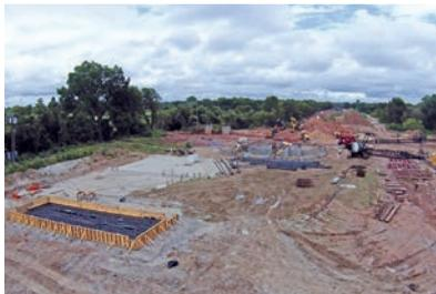
The new WMARSS Transfer Lift Station is well underway. The project involves building a completely new lift station facility, bypassing and removing the La Salle Ave. Lift Station, improved odor control, and the installation of a new forcemain to the central wastewater treatment plant.
