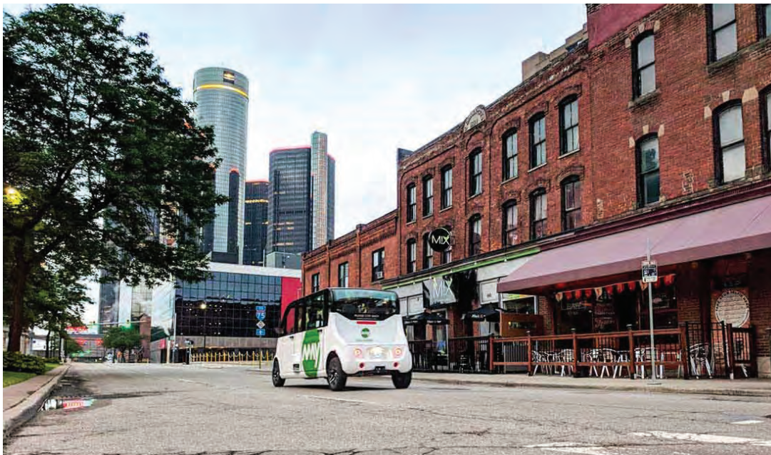
Figure 5.4. Cities might partner with autonomous shuttle providers to maintain efficient service in certain locations (May Mobility)
