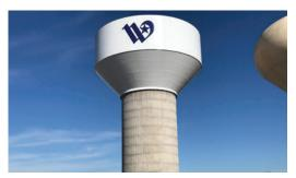
The new Ritchie Road Tower, at Ritchie Rd. and Panther Way, is complete and fully operational. The new two-million-gallon composite tank replaces the previous, 33-year-old tank. Demolition and removal of the old tank is expected to be complete later this year.
