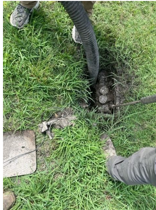
Vacuuming Out the Debris
