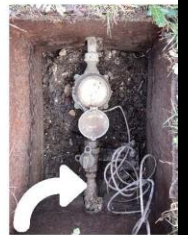
Replacing lead service lines like this one is part of the City of Waco Action Plan
