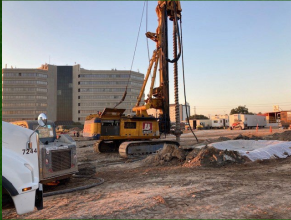
Auger Cast Pile Operations, October 2022
