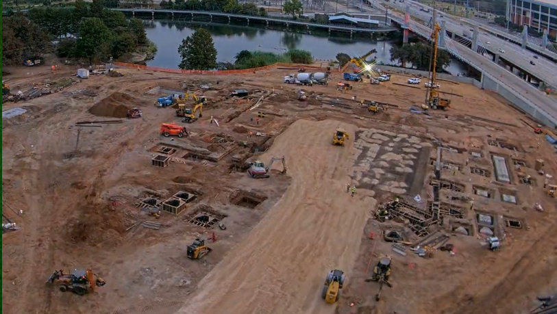
Concrete Foundations; Crane Pad Preparation, October 2022
