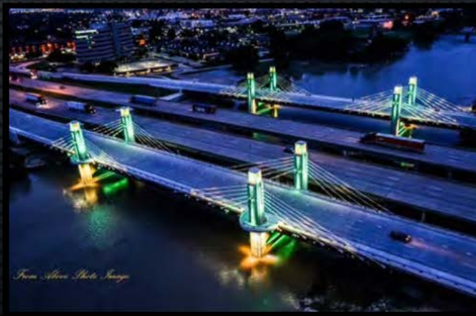
Multiple Column Bent – matches the “Art Deco” look of the Brazos River (BRG)
